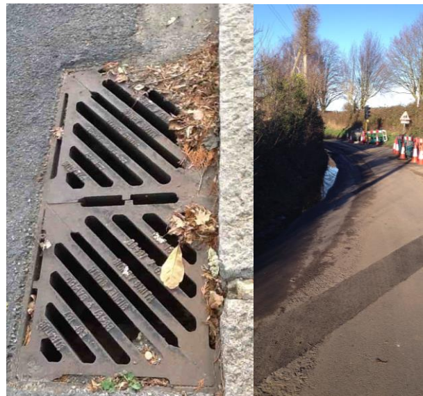
No action required: Intervention level not met
